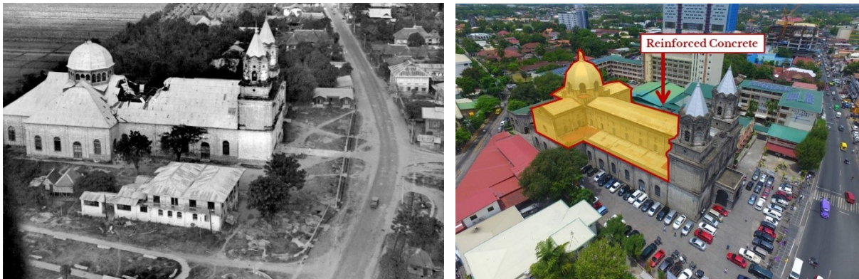
Image 1 Left photo: 1945 photo of the HRP, showing the gaping hole left by the war aircraft above the church's nave (Photo by © Robby Tangingco). Right photo: 2019 photo of the HRP. The superstructure made of reinforced concrete we see today was virtually non-existent in the original structure of the church (Photo by © ETFFI).
