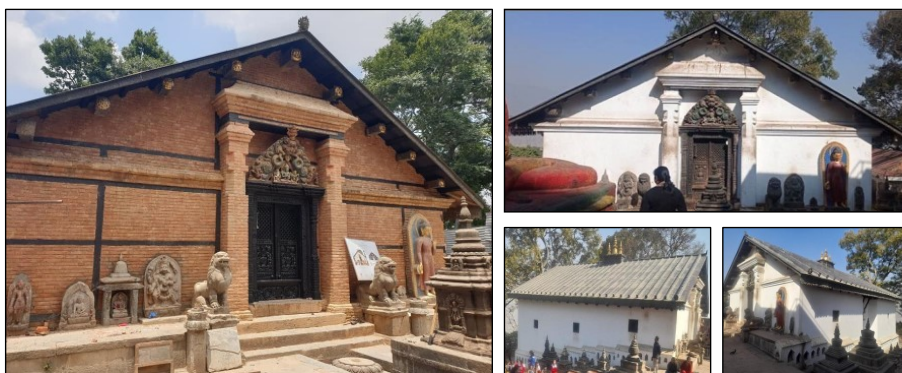
SHANTIPUR TEMPLE : After Rehabilitation
