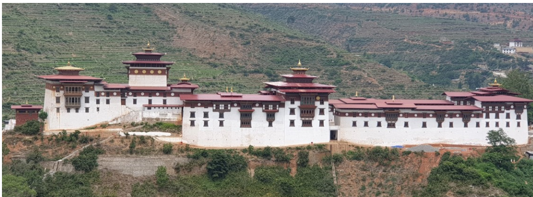
Figure 9. Dzong after Reconstruction. Source DCHS
