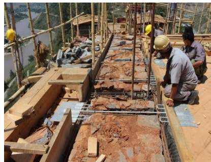
Figure 6. Installation of Wangdue latch Source: DCHS
