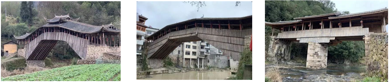
Figure 3. Xuezhai Bridge (left), Wenxing Bridge (middle) and Wenzhong Bridge (right) after reconstruction
