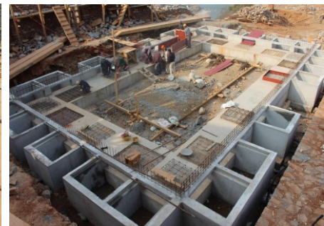
Figure 7. Construction of base isolation Source: DCHS
