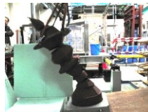
Inspection of antiseismic structure (The Noto Hanto Earthquake)
