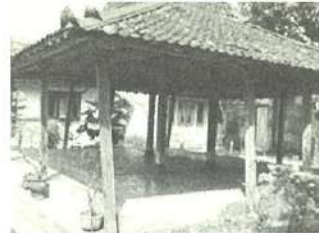
The twisted (muntir) soko rowo and soko guru. But the roof still stands.
