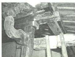
Bahu danyang (console) was corroded.
