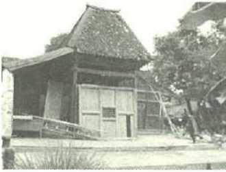
Dudur and blandar tritis (ring balk) was broken and caused the usuk, reng, and genteng (tile) slippage.
