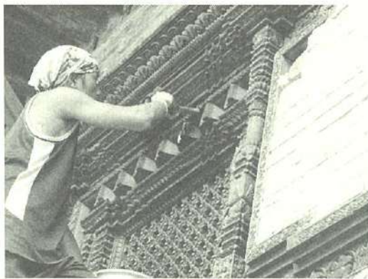
Figures 10, 11. Cleaning and applying a kerosene and linseed oil solution (Patan royal palace)
