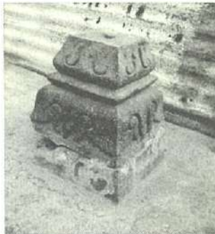
Displaced umpak (foundation). (photo: author)
