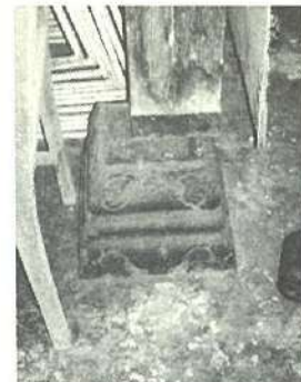
Soko guru and soko rowo (main and peripheral columns) displaced from their foundations because of the vertical and horizontal quake.
