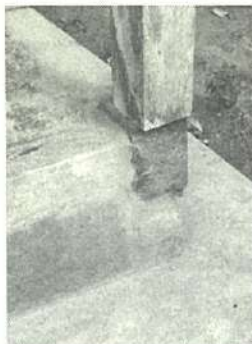
Soko guru and soko rowo (main and peripheral columns) displaced from their foundations because of the vertical and horizontal quake.
