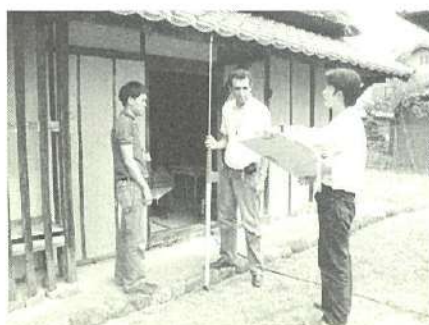
Drawing the elevation of the house by measuring
