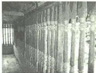
Lacquered timber railing and details of a stairway
