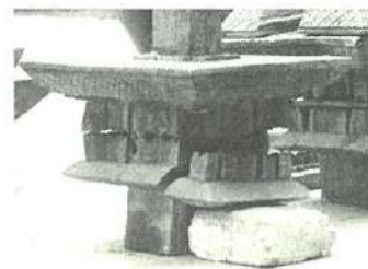
Untu walang , the connecting element between soko guru and sunduk , was broken.
