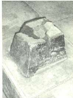
Broken umpak (foundation)
