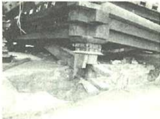
Sunduk pemanjang and penyelak as the key structure was broken.
