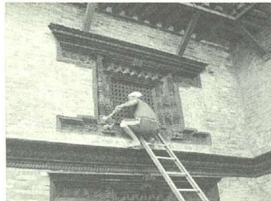
Figures 10, 11. Cleaning and applying a kerosene and linseed oil solution (Patan royal palace)
