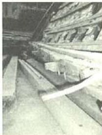
The steel plate in joglo lambang gantung slipped.
