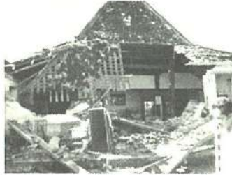
Dudur and blandar tritis (ring balk) was broken and caused the usuk, reng, and genteng (tile) slippage.
