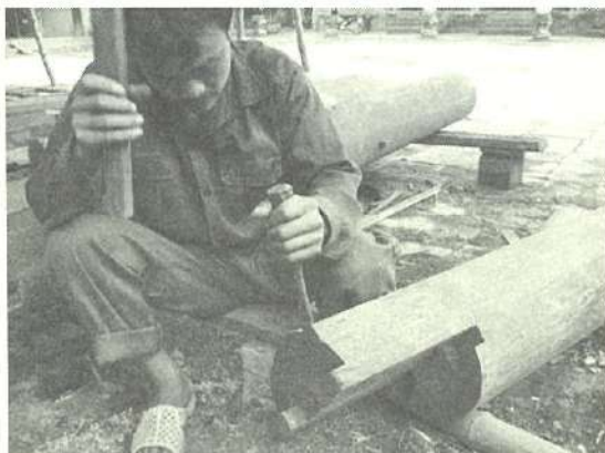
Picture 2. Joining a column
