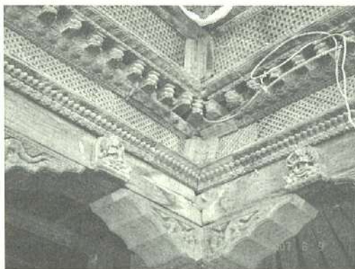
Figures 12, 13. Replacing old woodwork with new (55-Windowed Palace, Bhaktapur)
