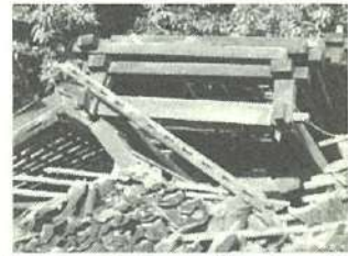
Soko guru broken, making the entire roof fall down. But the tumpang sari still rigid.
