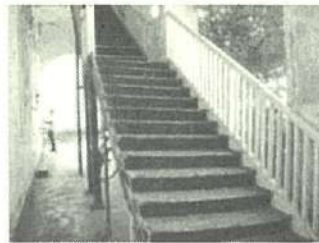
Lacquered timber railing and details of a stairway
