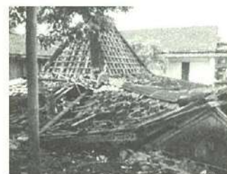
Soko guru broken, making the entire roof fall down.
