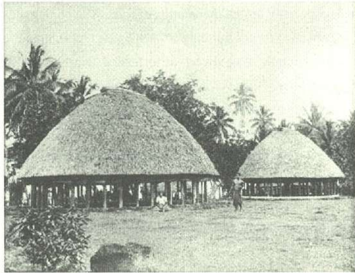
Houses complete with the floor covered with pebbles, and the blinds already done and being put up when the weather is hot.
