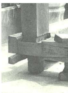
Pre-reconstruction with original material. The connection of sunduk-ktli and soko guru was broken.
