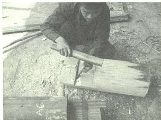
Picture 2. Joining a column
