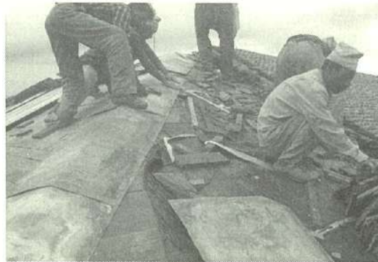
Figure 7. Roof tiles and planking in the roof of the 55-Windowed Palace, Bhaktapur
