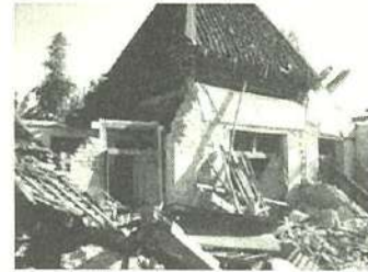
Dudur and blandar tritis (ring balk) was broken and caused the usuk, reng, and genteng (tile) slippage.
