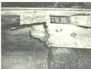
Connection between blandar (balk) broken by corrosion.
