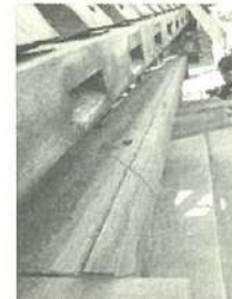
Takir slipped because of the small connection ( pasak ) fell away from its blandar (balk).
