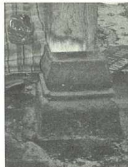
Soko guru and soko rowo (main and peripheral columns) displaced from their foundations because of the vertical and horizontal quake.
