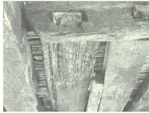
Mortise and Tenon method of assemblage
