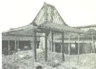
All of soko rowo (peripheral column) collapsed, but the roof still stands with only the four soko guru (main column)
