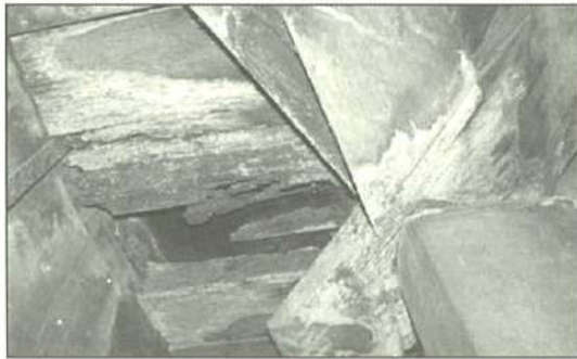
Damaged wooden structure of the Trayodasha Bhuvana
