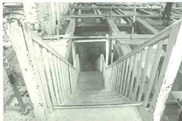
Figure 33: Decayed wooden stair
