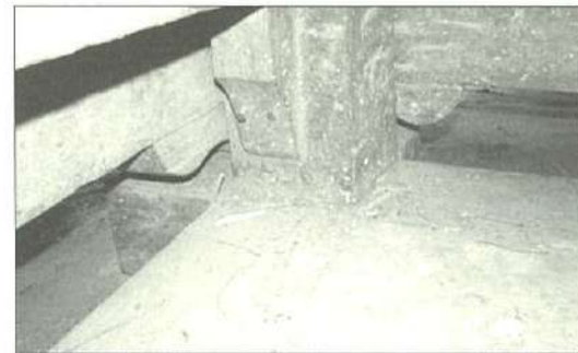
Wooden structure damaged by bird droppings (now cleaned)
