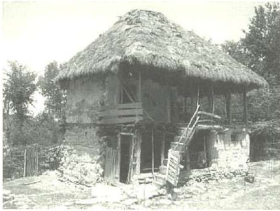
Photo 34: Construction with zogmei walls in the western foothills area (Tarabi's house)
