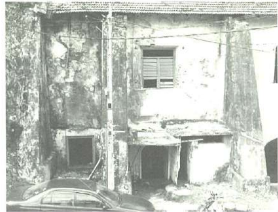
Figure 21: Damage to the wall
