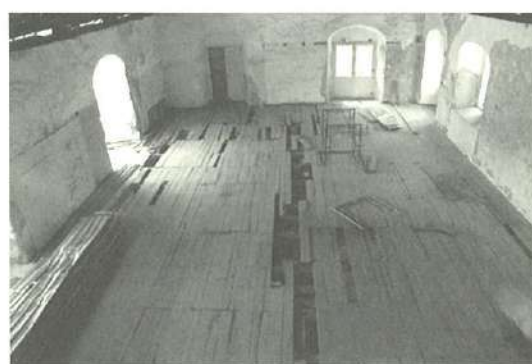
Figure 26: Damaged timber floor
