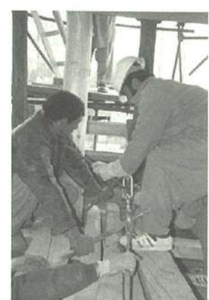
Fig. 38. Turning buckles being used to pull back the tilted loggia
