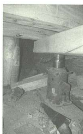
Fig. 37. Lifting the loggia to a stable state with the help of hydraulic jacks
