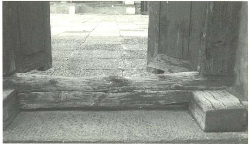
Deterioration of a doorstep
