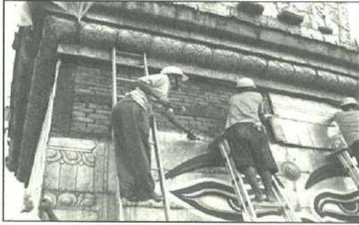
Removing copper sheets from the Hermika
