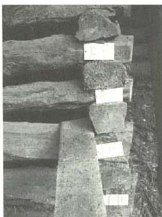
Photos 17 -19: Method of laying zogmei wall beams over each other
