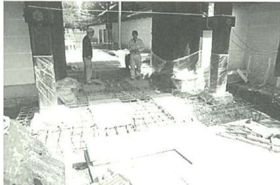
Fig. 12 Use of reinforced concrete under a gate
