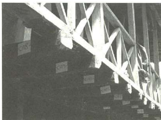
Photo 80: Labeling the columns of the first floor
