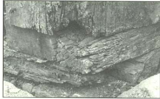
Deteriorated wooden members in the Hermika
