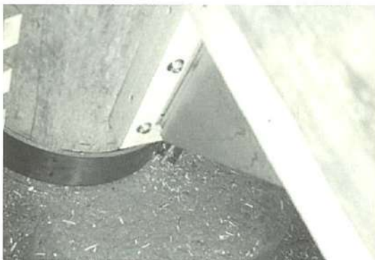
Fig. 13 Earthquake resistant device on the column base
