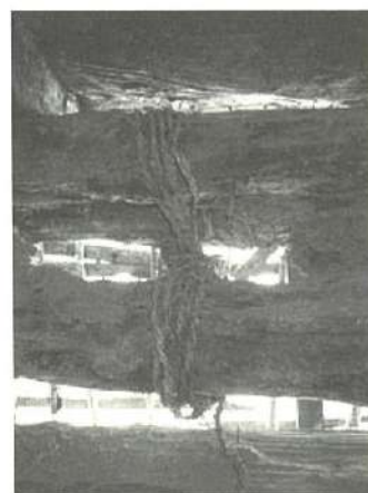
Photos 17 -19: Method of laying zogmei wall beams over each other
