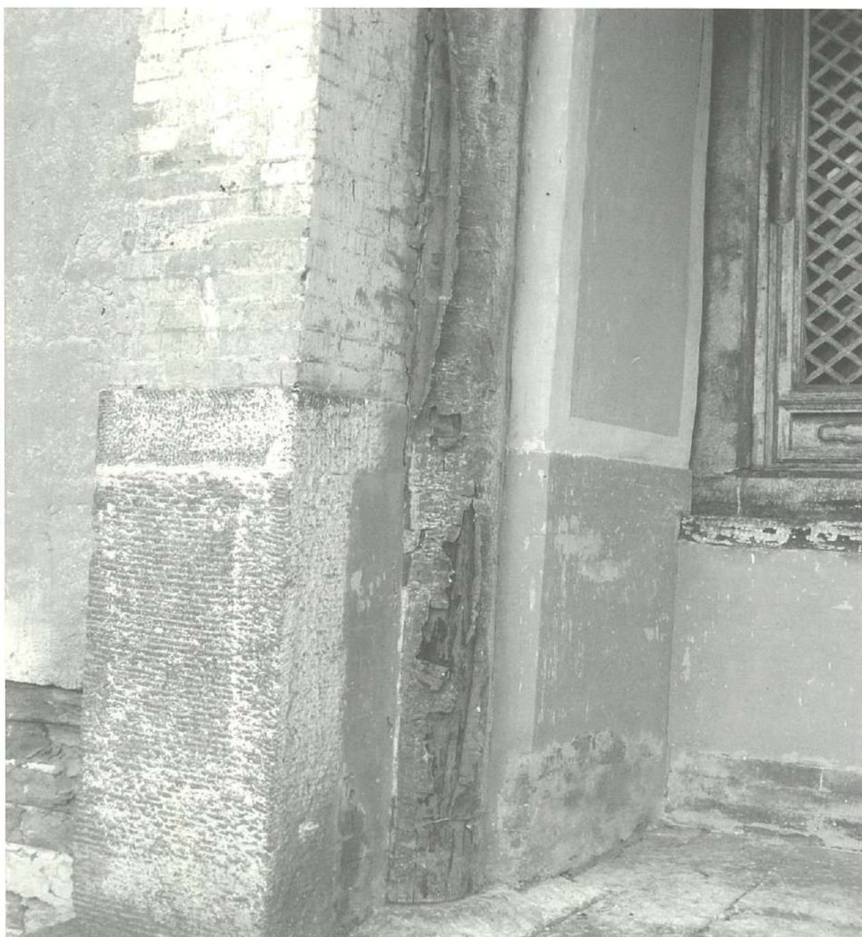
Column of the Amarbaysgalant monastery. The coating of paint was peeling away, and some parts of it were missing.
