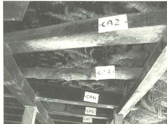
Photo 79: Labeling the beams of the first floor
