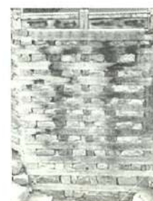
Fig 14. Detail of cator and cribbage in the entrance loggia of Khaplu palace
