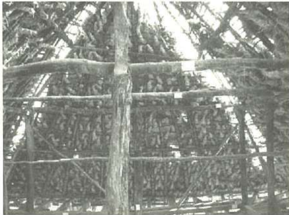
Photo 78: Labeling the truss of a sloping roof
