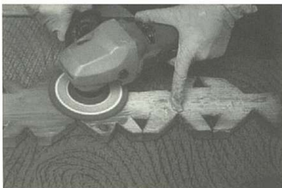
Photos 74 - 75: Cleaning and renovating the rails
