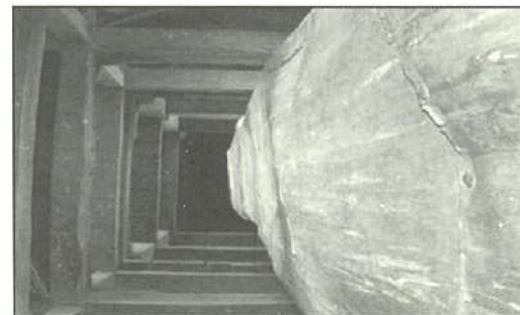
The central backbone “Yashthi” of the stupa
