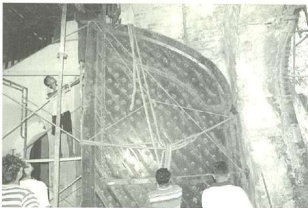
Figure 30: Dismantling of the door
