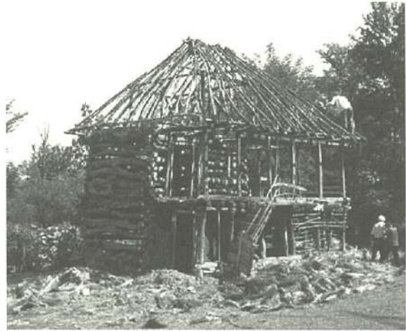
Photo 35: Tarabi's house, displaying the wooden frame
