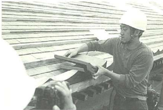
Fig. 11 Demonstration of tile fixing on the roof
