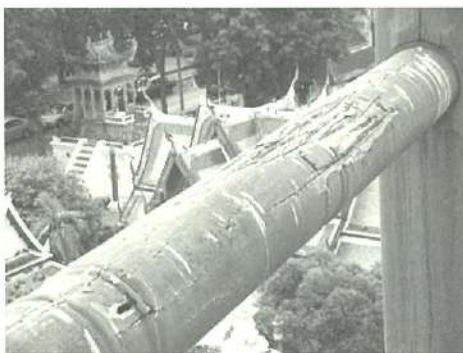
Deterioration of the wooden structure
