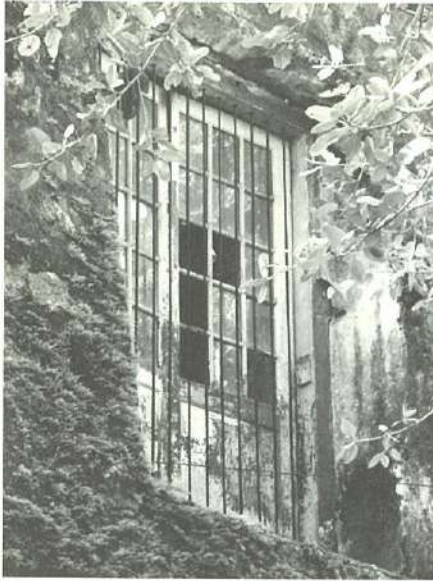
Figure 27: Deterioration of a window
