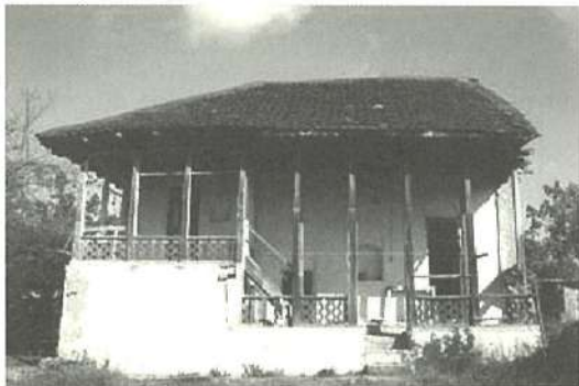
Photo 33: Building with mud and sun-dried brick walls in the western plain (Moosazadeh's house)
