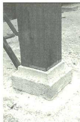
Figure 14: Insulation against dampness and insect attacks
