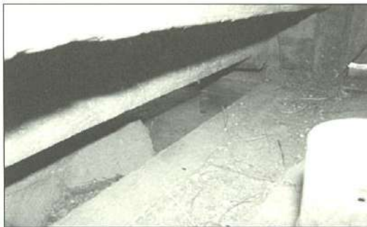
Wooden structure damaged by bird droppings (now cleaned)
