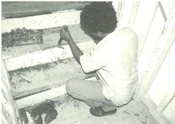
Figure 34: Removing decayed parts
