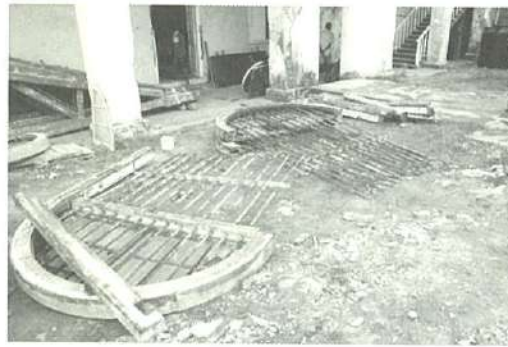
Figure 28: Replacing of decayed parts
