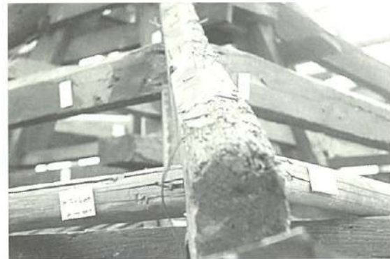
Fig. 20 Numbering of wooden roof elements completed
