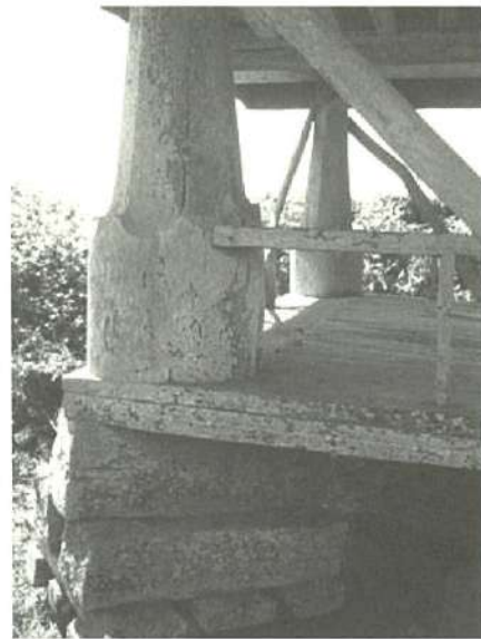
Photos 26 - 27: Rice storeroom constructed over a well-shaped base
