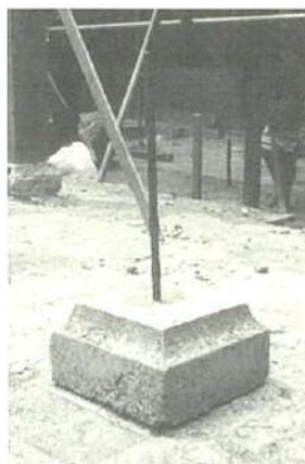
Figure 14: Insulation against dampness and insect attacks
