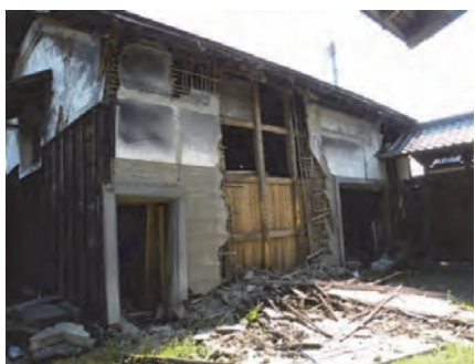
写真8 土蔵の被害状況 Photo 8. Damaged condition of a storehouse
