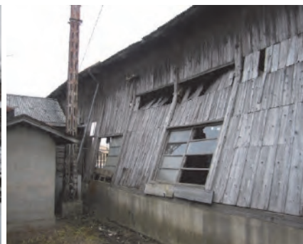
写真5 柱の折損 Photo 5. Damaged pillars
