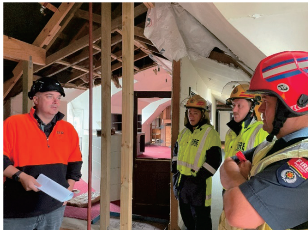
Figure 9. Local fire crew and fire protection systems provider visiting former Provincial Council Buildings, early 2023. Photograph: Amanda Ohs
