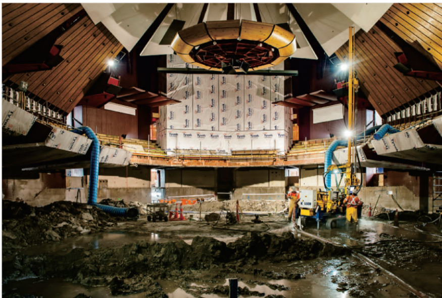
Figure 11. Christchurch Town Hall auditorium, ground remediation works. Photograph: CCC collection
