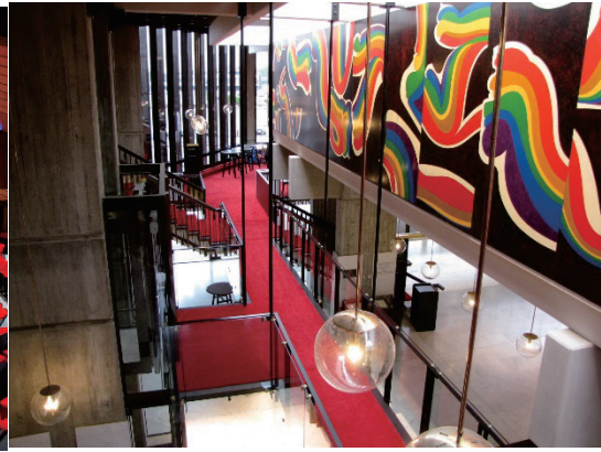
Figure 14. Christchurch Town Hall foyer, reinstated heritage fabric. Photograph: CCC collection
