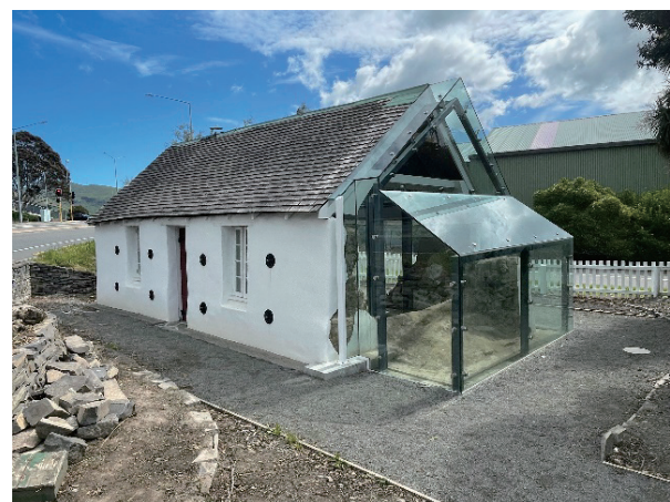
Figures 3, 3a. Captain Penfold's Cottage repair and strengthening. The glazed build out reflects the form of the original chimney. Photograph: Deborah Cosgrove, November 2023.
