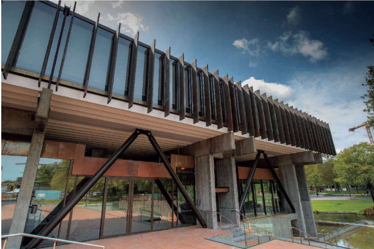
Figure 8. New Function Room (below) with new structural supports and rebuilt columns for the Limes Room (above). Christchurch City Council, 2019
