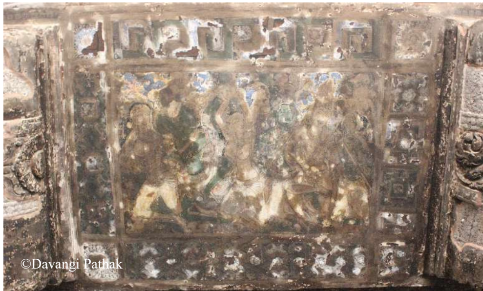
Deterioration of a wall painting on the ceiling of Cave no. 32, depicting celestial beings dancing and singing
