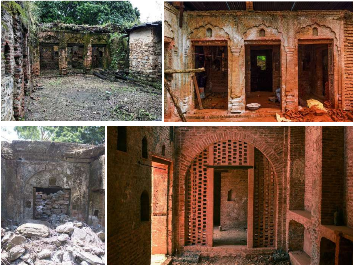
Images of a historic structure before (Left) and during restoration (Right), belonging to a private stakeholder. Image Credits: Author
