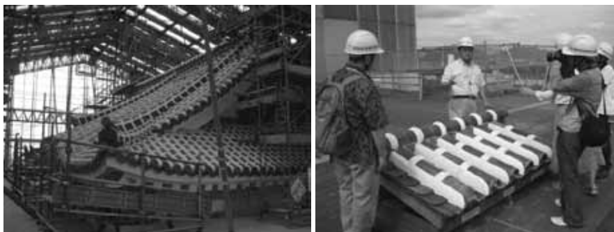
Figure 3. Left: Himeji-jo Castle restoration; Right: Research to find suitable roof plaster
