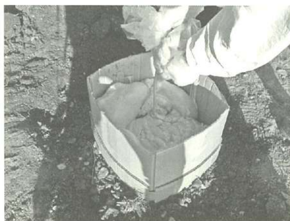
Urethane foams and solidifies to 10 times its original volume.
