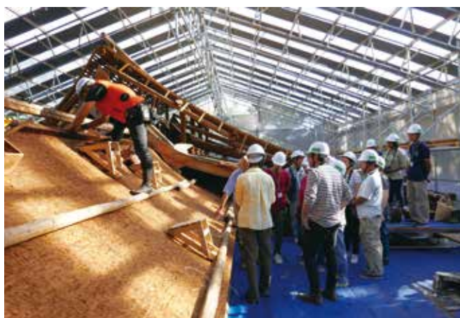
Roof restoration site at Yakushiji Yasumigaoka Hachiman Shrine (roof material: cypress bark)
