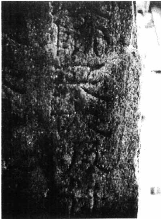
(Photo 9) Inscription after filling joint and defect
