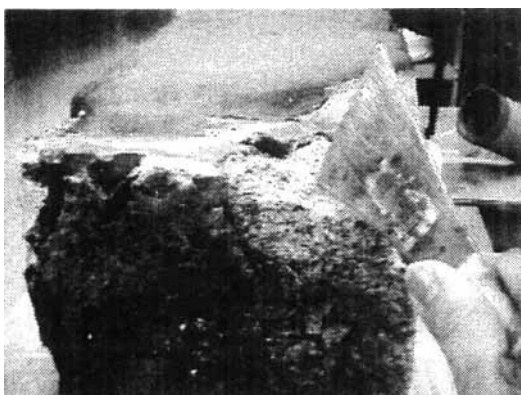
(Photo 12) Removal of filling material applied before
