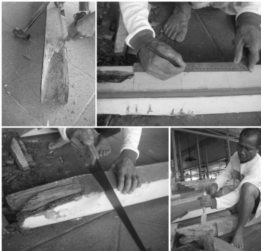
Replacing roof trestlework: (*top left*) identifying damaged parts, (*top right*) measuring to remove the damaged wood, (*bottom*) removing the damaged wood
