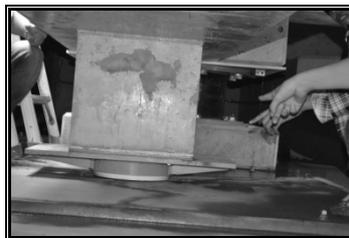
Installation of an earthquake resistant foundation at a traditional Kobe sake maker (*photo: Nikko Suko*)
