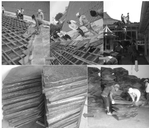
Dismantling the shingle roof after registration is completed
