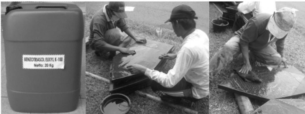
Using benzotriazole for conserving the copper plating on the original shingles
