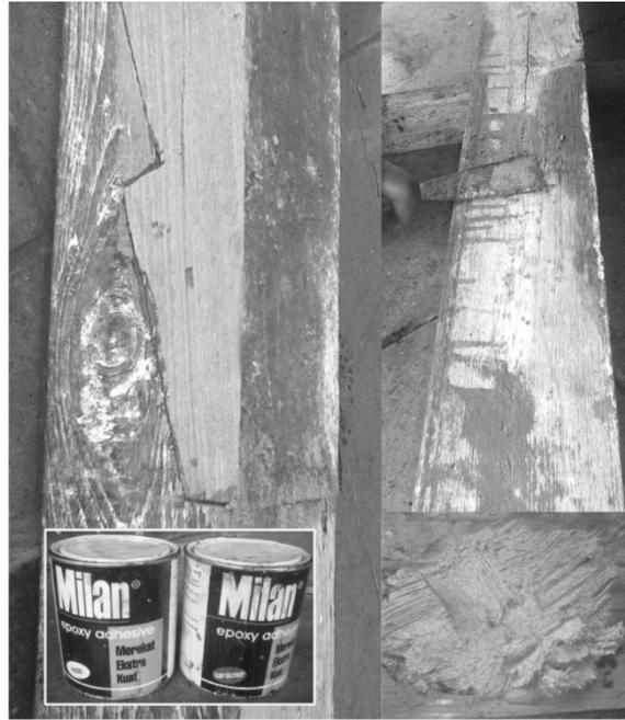
The original wood is glued together with new wood using epoxy, then the connection is camouflaged with wood putty.
