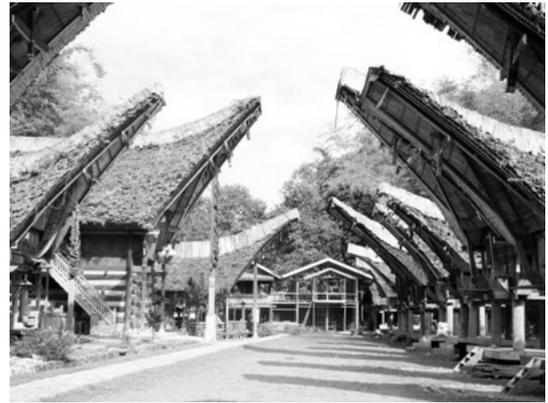
*Tongkonan* used bamboo and thatch for the roof covering
