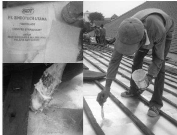
Fiberglass coating to cover cracks in the galvalume and to prevent further leakage
