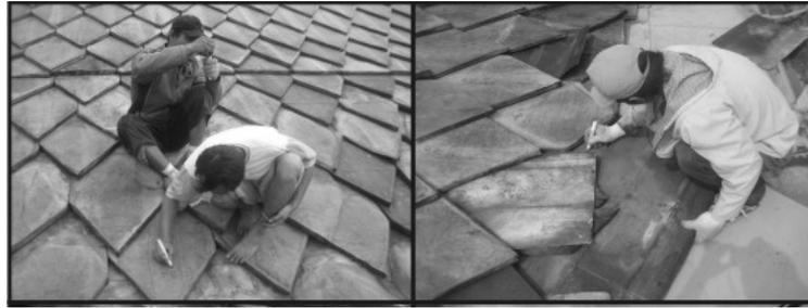
Numbering the shingles prior to dismantling
