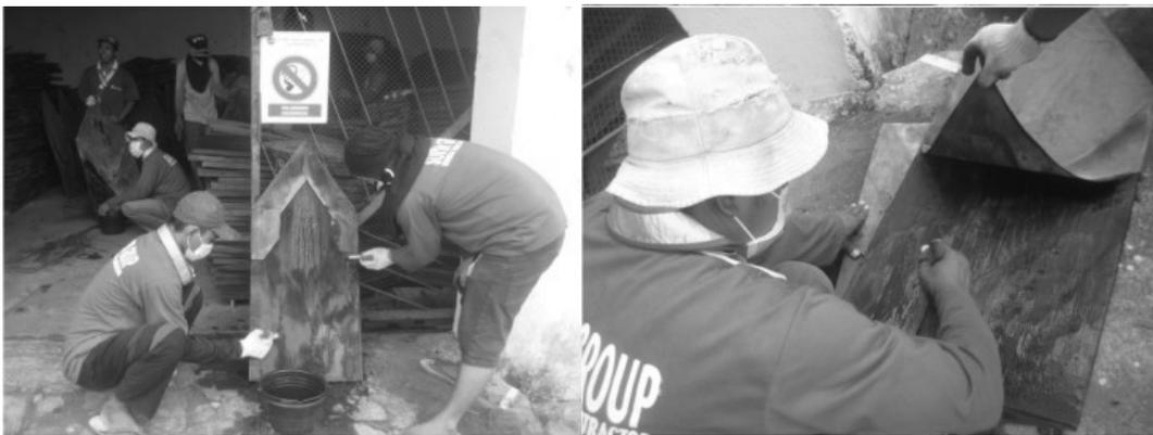
Application of chemicals to both sides of the original shingles, to prevent damage from termites
