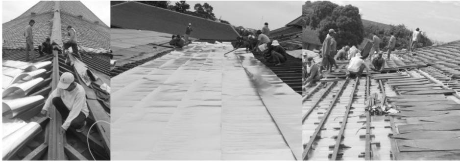
Installation of galvalume as a roof coating. Galvalume is used as a thermal barrier (insulator) and to prevent leakage. After the roof coating is laid, wooden ribs for the shingles are reinstalled.
