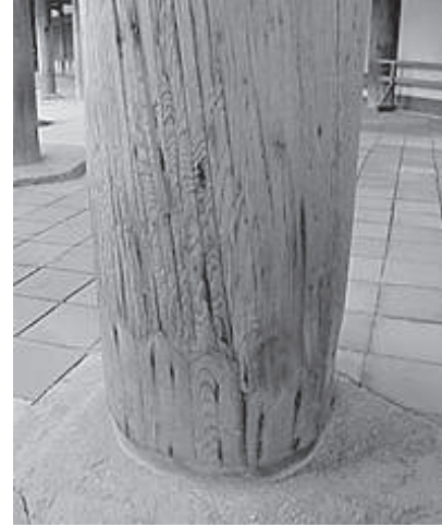
Fig.5: Replacement of decayed member
