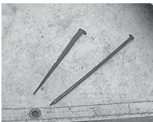
Fig.8: Varieties of nails used in different eras roof members being replaced
