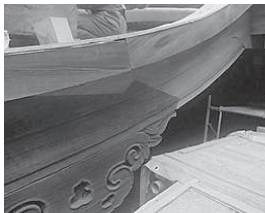
Fig.7: Joinery of old and new timber components
