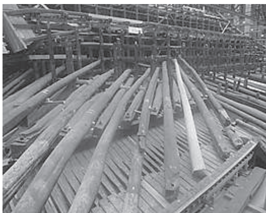
Fig.6: Decayed roof members being replaced roof members being replaced
