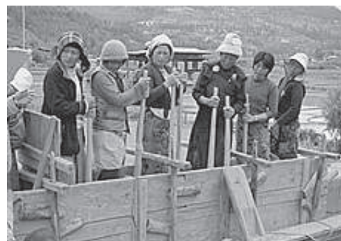
Fig. Rammed earth construction technique
