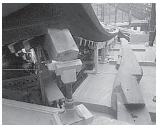
Fig.9: Eaves being jacked up to their original place
